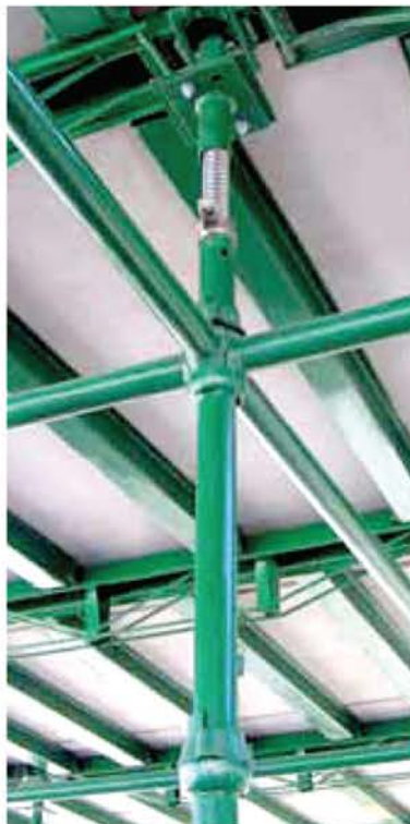
Decking Beam Size: 0.50 Mtr-1.70 Mtr
