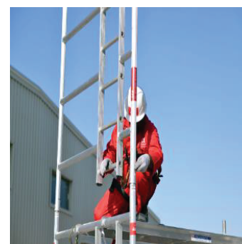
6 Fix the snap pin in order to lock the two frames and repeat the same for all frames.
