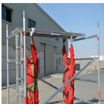
4 Fit the plain platforms on the top brace of the last frame.
